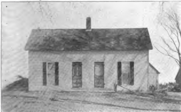
Residence of E. H. Burton, near Millard
